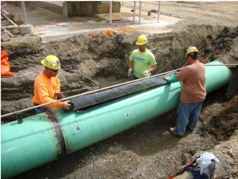
Figure 4: Precutting tape for cigarette wrap (Section 4.5.2)
